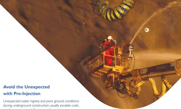
Unexpected water ingress and poor ground conditions during underground construction usually escalate costs, can have a negative influence on the environment, and inevitably cause significant delays. To counteract these risks, an economical approach is to pre-inject the ground ahead of the advancing face to avoid water ingress occurring, and to stabilize the ground.
