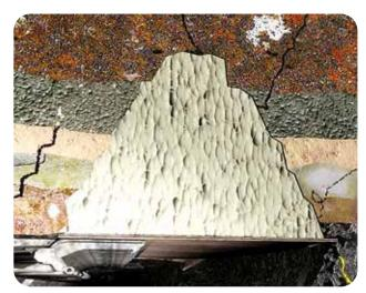
Cavity filling with MasterRoc® MP 367 Foam
