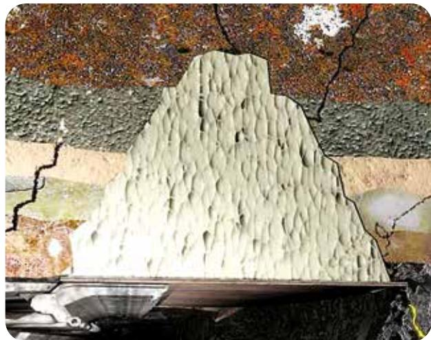
Cavity filling with MasterRoc® MP 367 Foam
