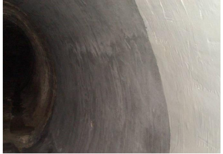
Concrete repair and protective waterproofing work on the gallery
