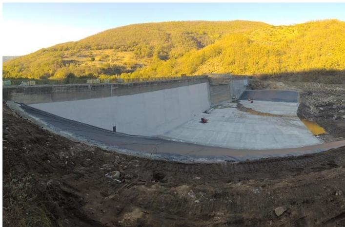
Application of MasterEmaco S 5300 medium modulus repair mortar and finishing with MasterSeal 6100 FX cementitious waterproofing membrane.
