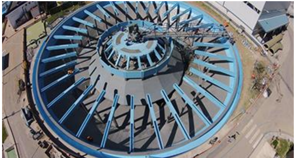
Aerial view of the primary sedimentation tank at the water treatment works ETAP El Atabal, (Málaga – Spain)
