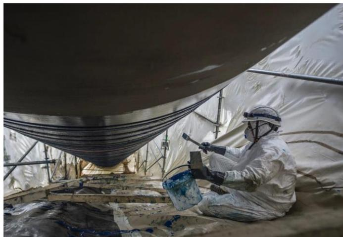
Application of MasterBrace carbon fiber to a penstock at EDF La Coche
