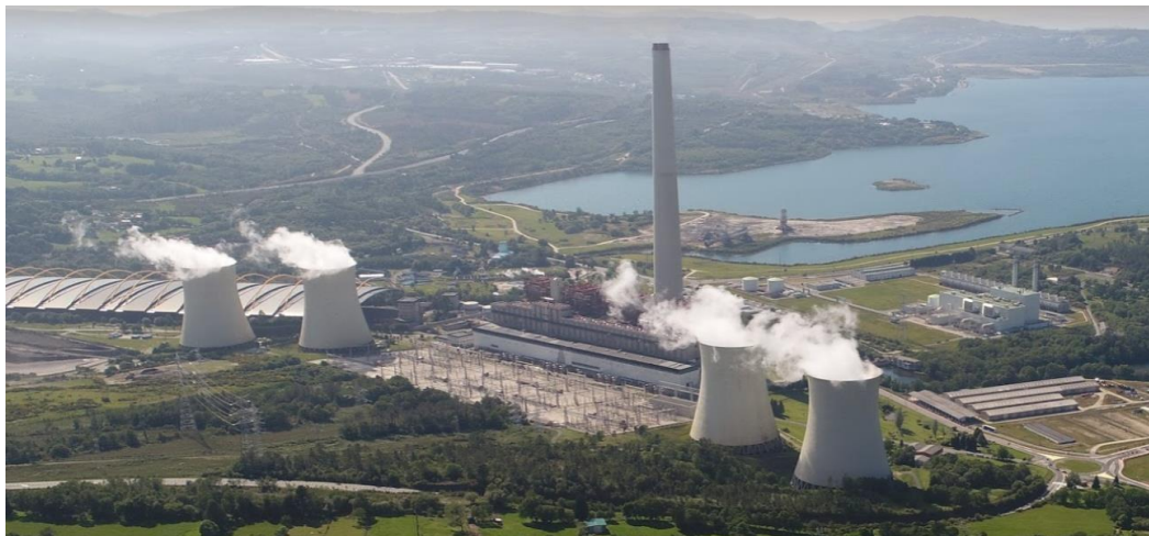
General view of the thermal power plant
