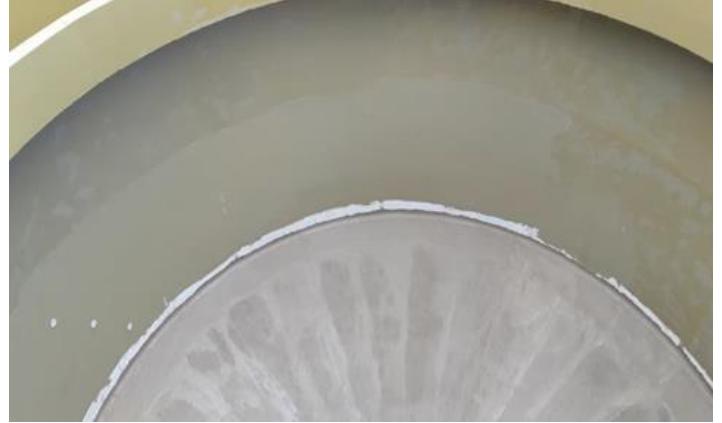
Tank application MasterSeal 7000 CR.
