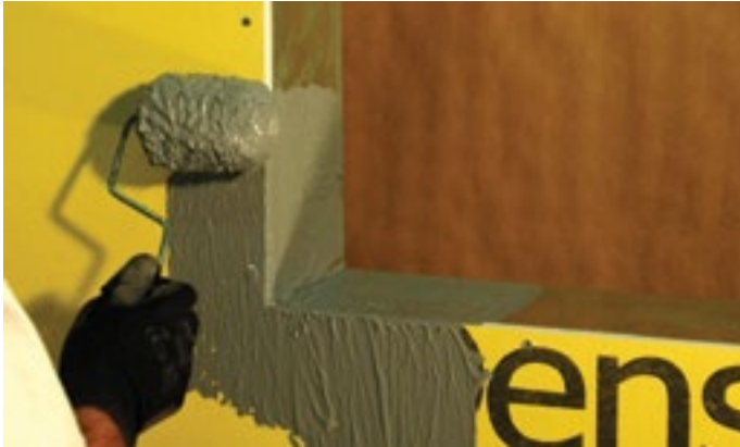
Step 1 Liberal apply fluid-applied BASF air/water-resistive barrier material.
