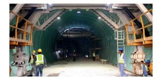
MasterRoc WP 1700: Synthetic plasticized PVC membrane for horizontal and vertical waterproofing MasterRoc WP 1950: PVC waterstop for construction joints treatment and compartmentalization MasterRoc WP 1780: Re-Injectable hose system for sealing construction and cold joints
