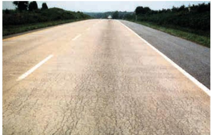
Figure 1. ASR-Induced Map Cracking in Pavement
