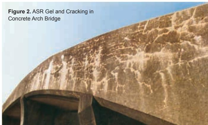
Figure 2. ASR Gel and Cracking in Concrete Arch Bridge
