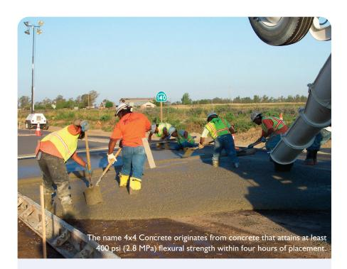
General contractor, W. Jaxson Baker Inc., was challenged with replacing an entire asphalt intersection with concrete within one week. The challenge was issued by CalTrans to minimize disruption to traffic flow and lane closures.
