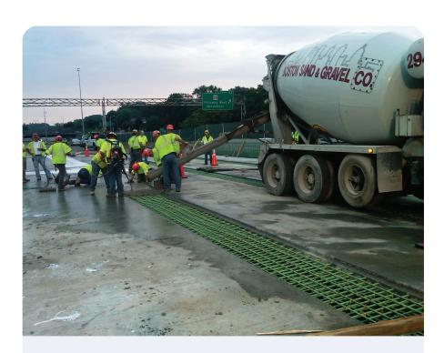
A total of 14 bridges on Interstate 93, where the traffic volume is 200,000 cars per day, needed replacement due to deterioration of the concrete. Using normal construction procedures, this project would have taken at least five years to complete.
