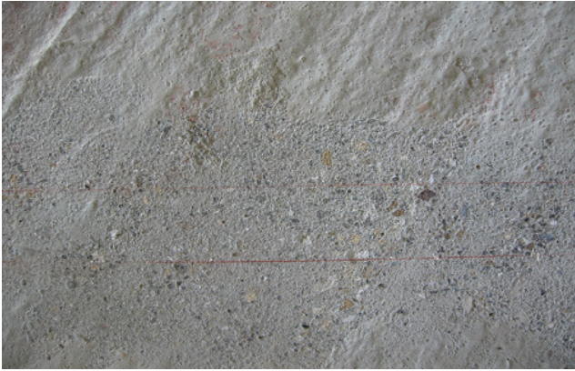
Figure 1. Grinded concrete surface prior to adhesive application.
