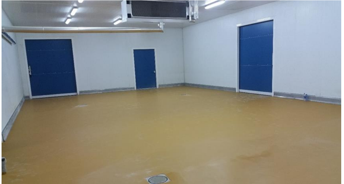
Our reference Ogun (Nigeria): Cormart Factory
