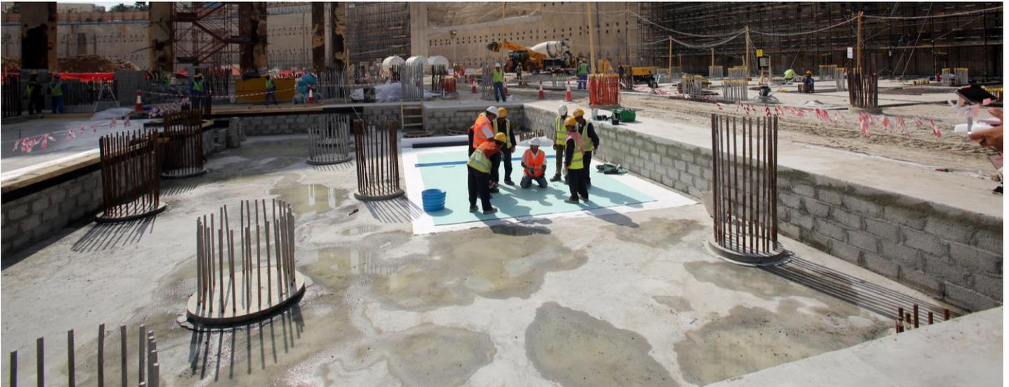
Waterproofing is often required for structures built at below ground level. Waterproofing considerations are especially important where ground water is likely to build up in the soil and raise the water table.
