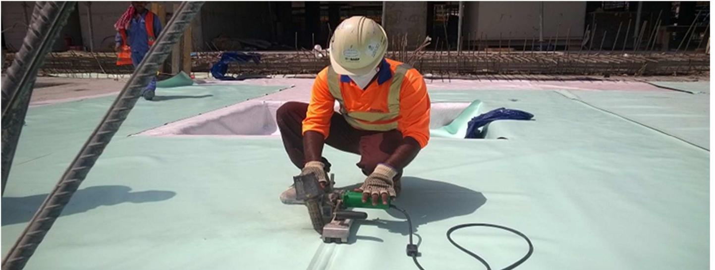
The issue of welding synthetic membrane seams (PVC / TPO) continues to be a concern when installing synthetic membranes. Plastic welding is a very technical operation which requires expertise by the installer and vigilance on the part of the Quality Assurance monitor. When a waterproofing system leaks, 9 time out of 10, the product manufacturer, product or equipment usually get the blame, when often the problem is the poor installation or welding of the system.
