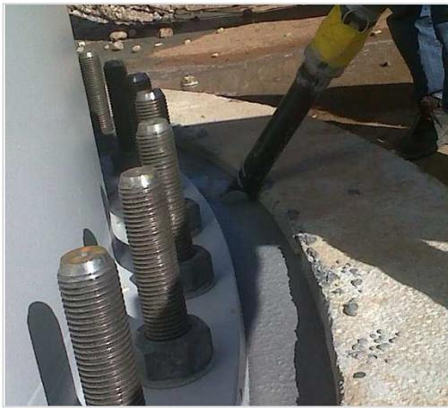
**Grout (Webster):** A thin mortar used in filling joints and voids fluid enough to be poured.
