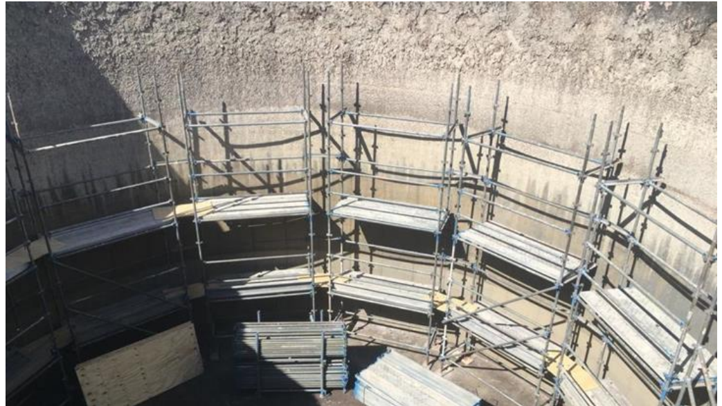
Our reference in Boxtel, Netherlands: repair of a buffer tank
