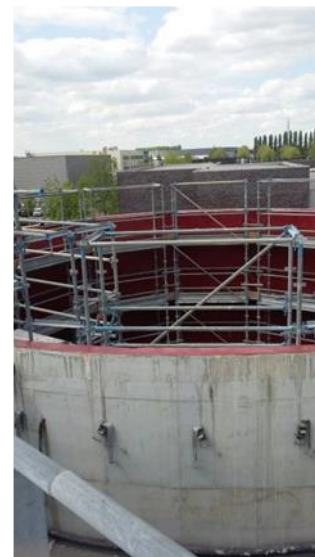
Our reference project at Vion, Netherlands: repair of a buffer tank.
