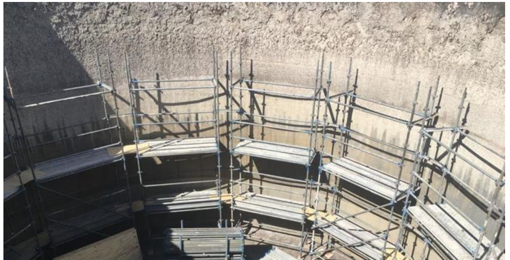
Our reference in Boxtel, Netherlands: repair of a buffer tank
