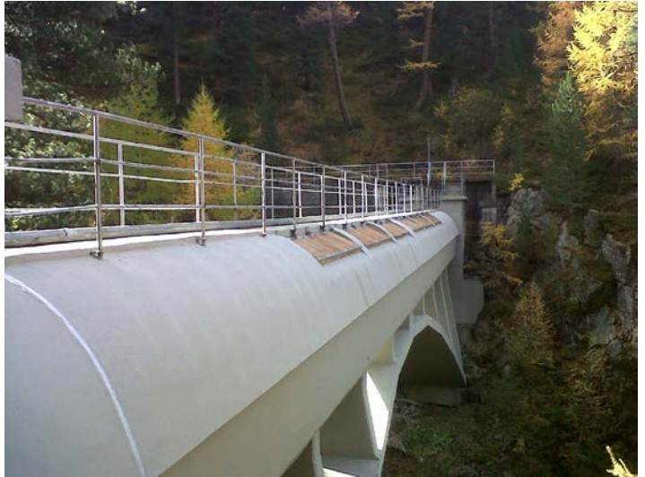
Our reference in Livigno (Italy): Waterproofing of bridge channels Tresenda and Vago
