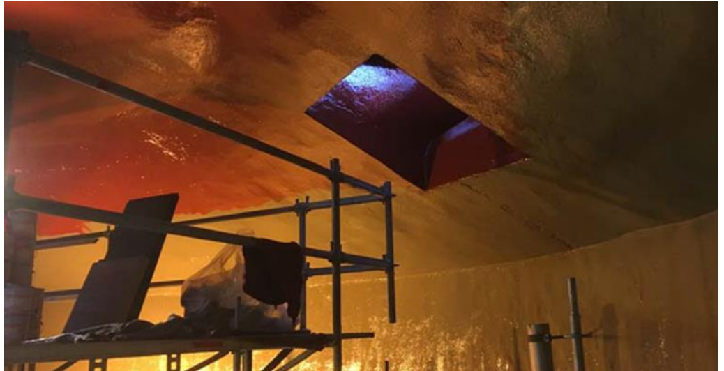
Digester renovated with MasterSeal 7000 CR, (Kongens Lyngby - Denmark)
