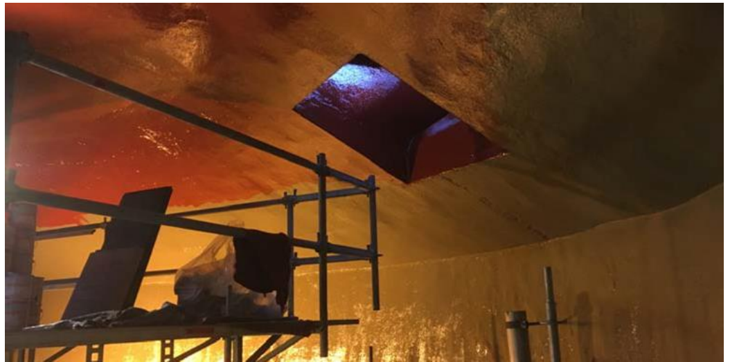
Digester renovated with MasterSeal 7000 CR, (Kongens Lyngby - Denmark)
