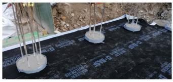
MasterLife WP 754 RT is cut and feathered to wrap around the pile cap joining the MasterLife WP 754 membrane to the pile cap and creating a fully bonded area. The excess is cut and folded onto the top of the pile cap.
