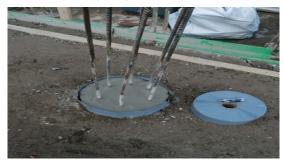
MasterLife WP 754 membrane is cut slightly inside the pile cap dimensions allowing for a 20mm overlap once the membrane is pulled over the pile cap to the base.
