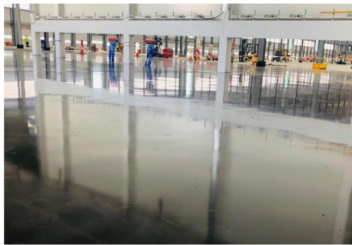
Our reference in Euro Central Business Park (Central Scotland): LIDL UK Distribution Centre
