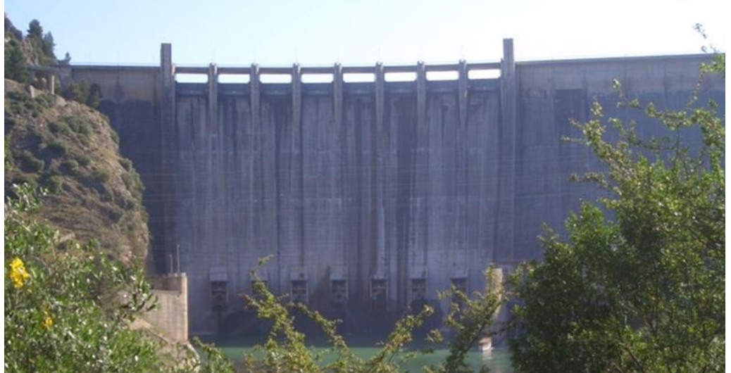
View of the Iznájar dam in Córdoba (Spain)
