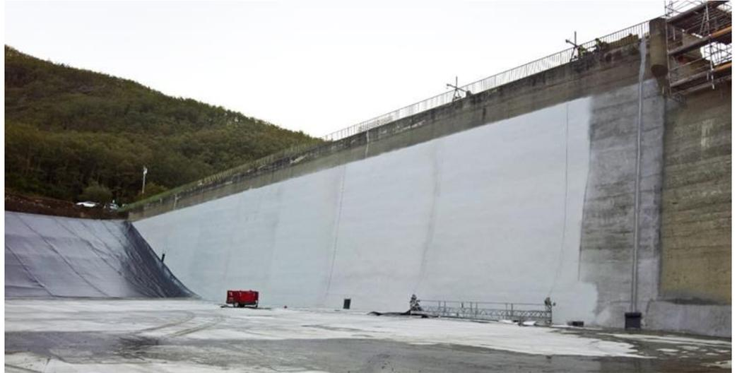
Concrete refurbishment on the upstream face of the dam. Presa de Horcajo in Hervás-Cáceres (Spain)
