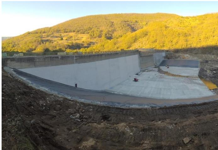
Application of MasterEmaco S 5300 medium modulus repair mortar and finishing with MasterSeal 6100 FX cementitious waterproofing membrane.
