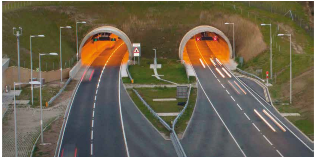
Our reference in Surrey (United Kingdom): Hindhead Tunnel
