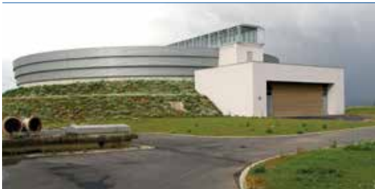
Tank for potable water
