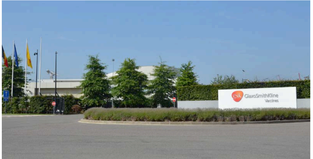
Our reference in Wavre (Belgium): Waterproofing and Protection of a Neutralization Basin
