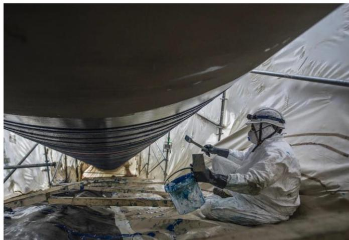
Application of MasterBrace carbon fiber to a penstock at EDF La Coche
