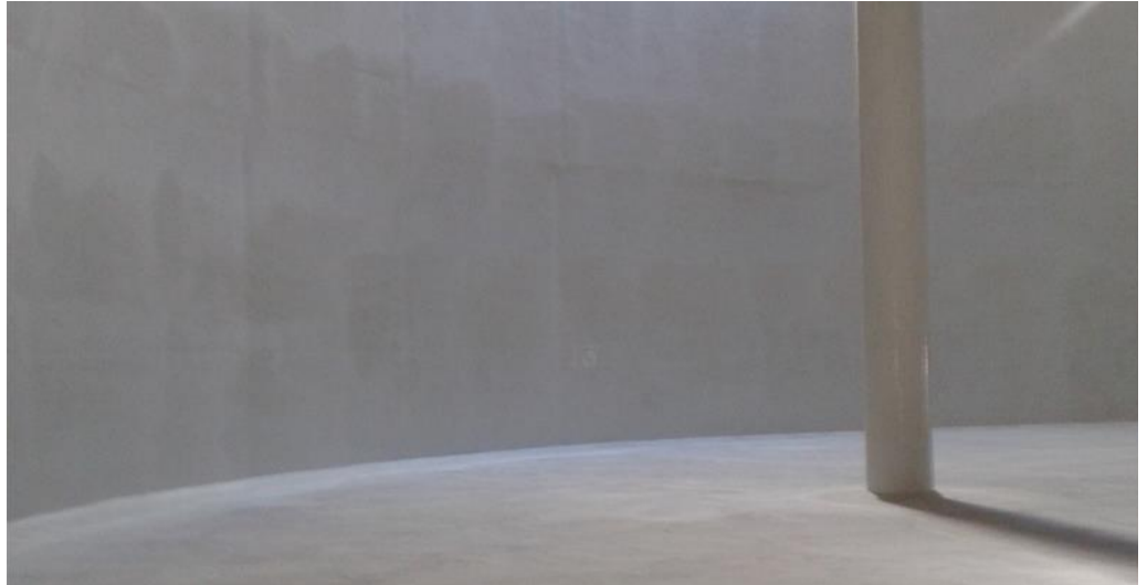
Our reference in Limassol (Cyprus): Waterproofing of potable water tanks
