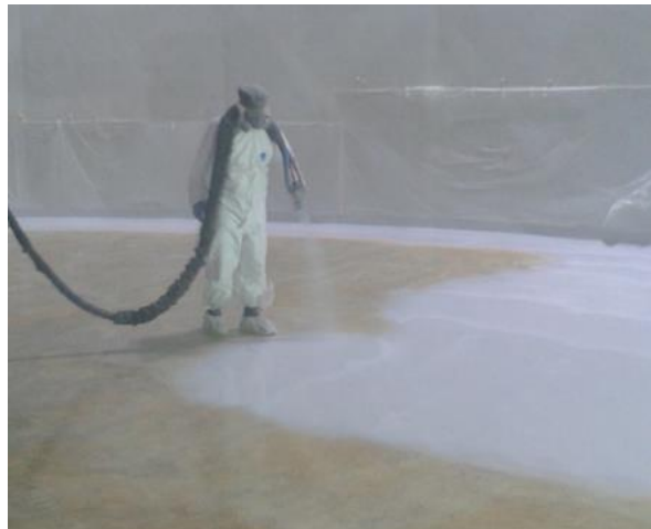
Application of MasterSeal M 689 polyurea waterproofing and protection membrane.
