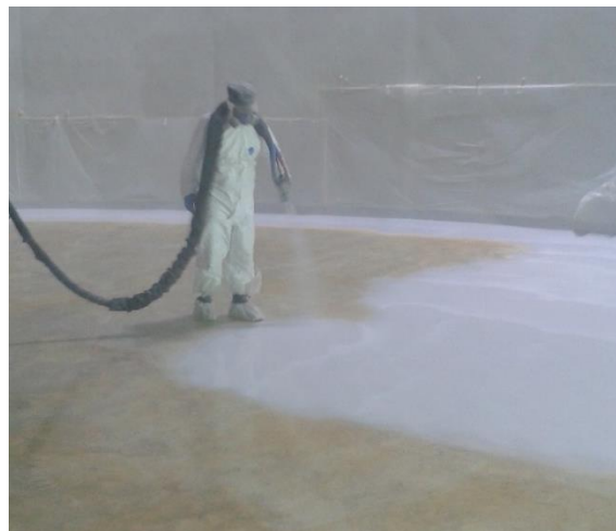
Application of MasterSeal M 689 polyurea waterproofing and protection membrane.
