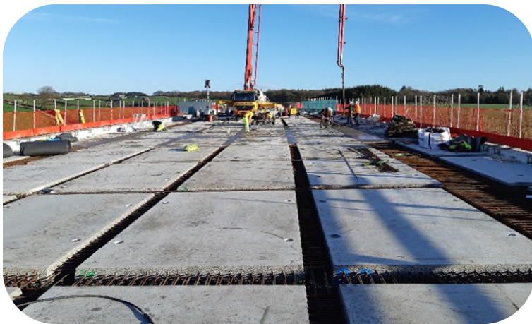
Our reference in North Ayrshire (United Kingdom): A737 Dalry Bypass
