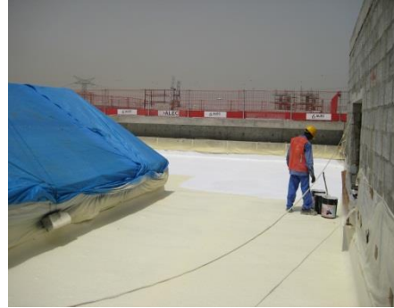
Applying MasterSeal® 550 (Dark Grey) two component, acrylic modified, flexible, Cementitious coating
