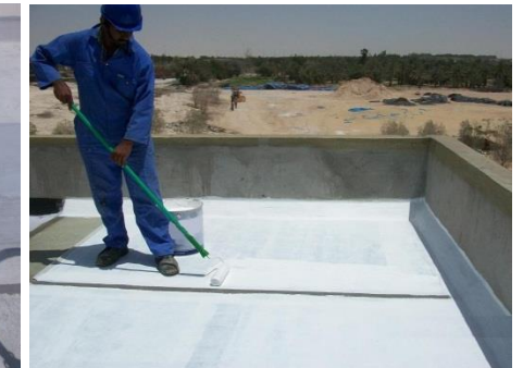
Joint Sealant & MasterSeal® 550 (White) final protective waterproofing coating
