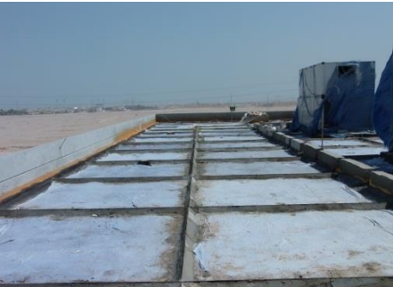
Water test & screed protection works
