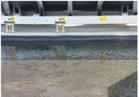
Applying MasterSeal® 550 (Dark Grey) two component, acrylic modified, flexible, Cementitious coating
