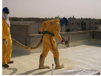
Elastospray® 1611/17 spray applied over the concrete slab
