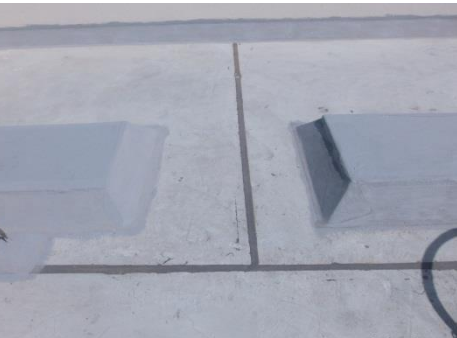
Joint Sealant & MasterSeal® 550 (White) final protective waterproofing coating
