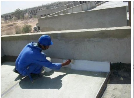
Joint Sealant & MasterSeal® 550 (White) final protective waterproofing coating
