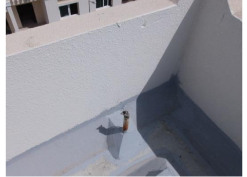
Applying MasterSeal® 550 (Dark Grey) two component, acrylic modified, flexible, Cementitious coating
