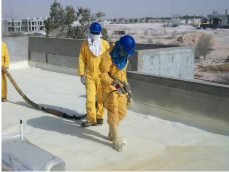
Applying MasterSeal® 550 (Dark Grey) two component, acrylic modified, flexible, Cementitious coating
