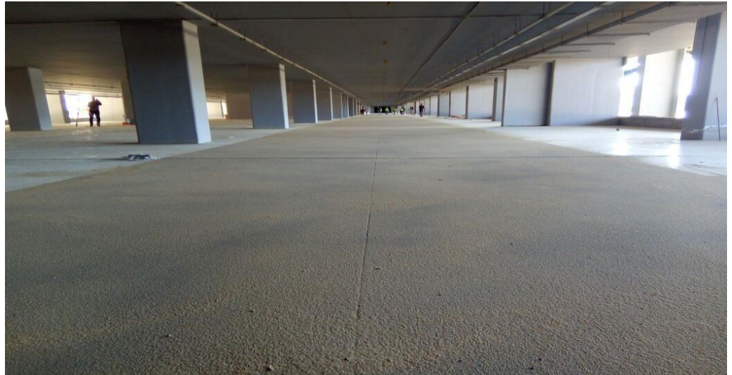
Our reference in Alexandria (Egypt): Sidi Gaber Bridge Car Park
