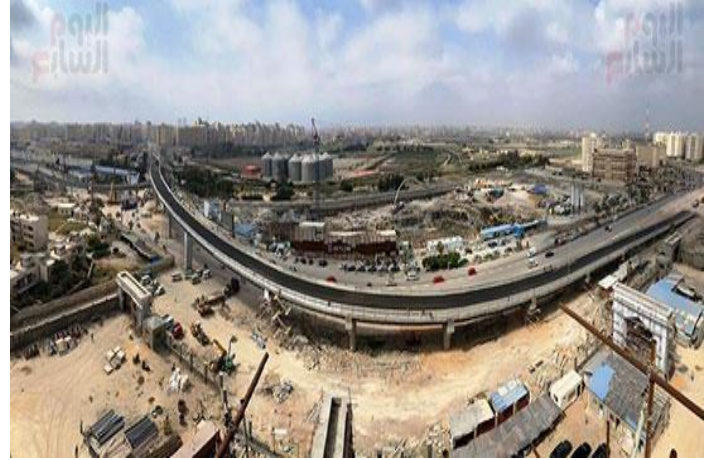
Our reference in Mahmoudia Corridor Bridges (Egypt): Alexandria
