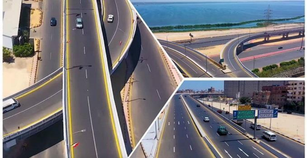
Our reference in Mahmoudia Corridor Bridges (Egypt): Alexandria
