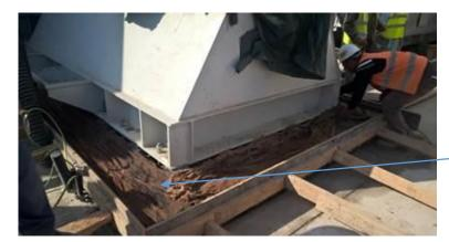
Saturate the concrete within the formwork with water for 24 hours
