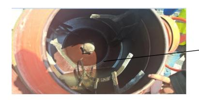
Flowable grout MasterFlow 524 will obtain that will pour through the upstand shutter with 45 degree that form the desired slope for grouting under this big machine
