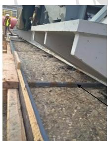
Fitted / tight wooden form work around the shoulders to prevent grout loss.
