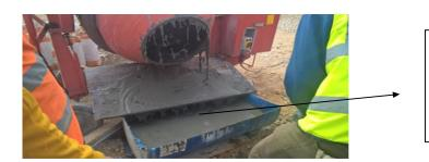
Adding 90% water the at beginning & then add the powder grout then mix for 1 minute then add 10% rest of water to have а good
