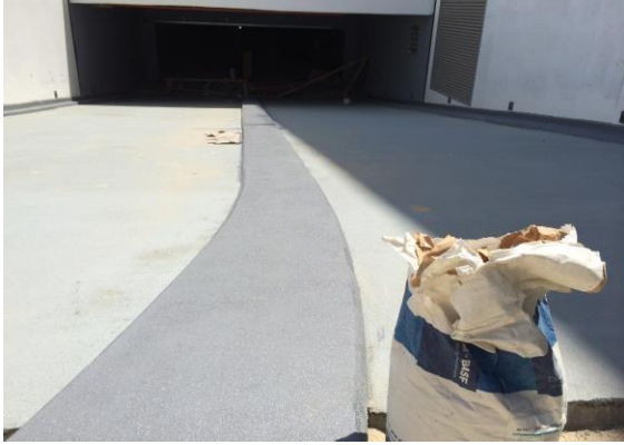
Epoxy Ramp System using ConiPur TC 458
