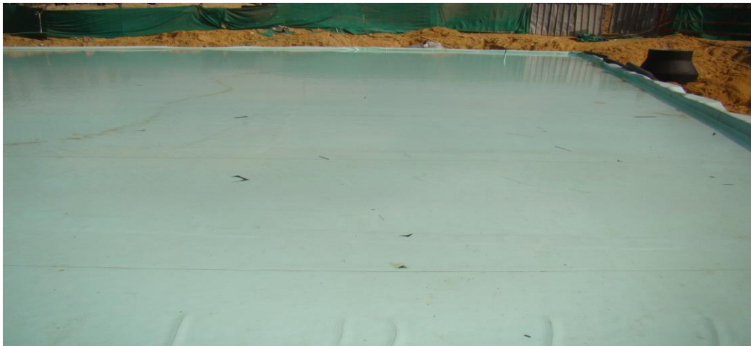
During Testing Master Builders Solutions PVC ( MasterPren BG 1.5mm )
