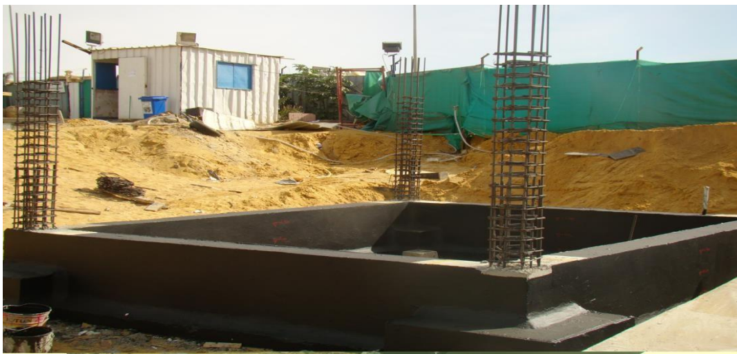
During Applying Damp Proofing product MasterSeal 622
