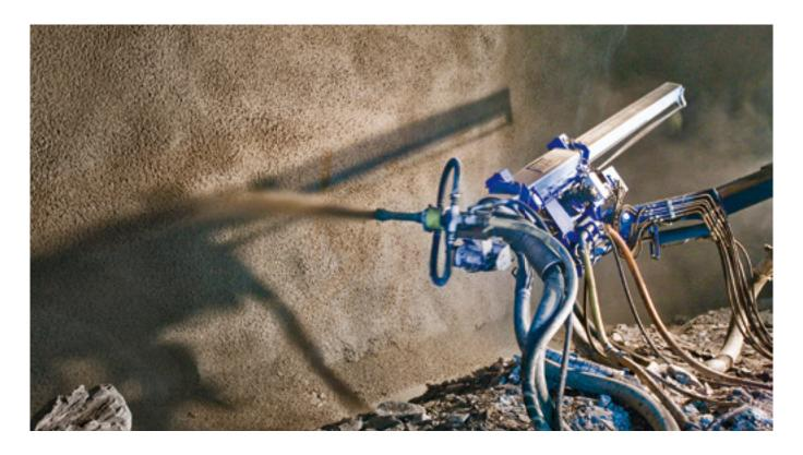
Sprayed concrete technology has revolutionized tunnel construction and mining operations since the middle of the 20th century. The development of material science and performance together with advances in spraying equipment technology have made sprayed concrete the building material of choice for today's underground construction projects.
