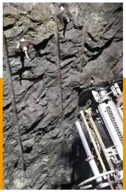
Self-drilling anchor with MasterRoc RBA 380
