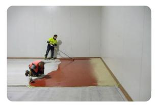
The concrete slab floor was first shot-blasted and had minor repairs made, prior to a 9mm thick trowel application of Ucrete DP 20
