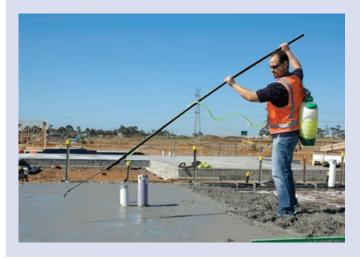
MasterKure 111 is especially effective in combating drying shrinkage cracking in hot weather concrete.
