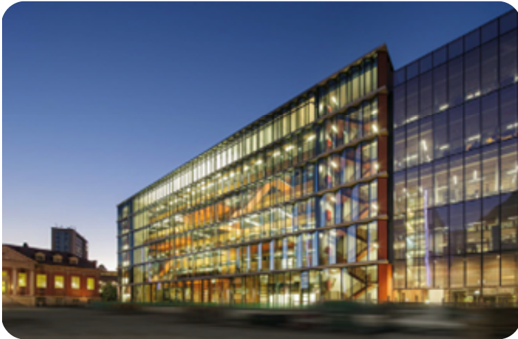
The Braggs Building, University of Adelaide
