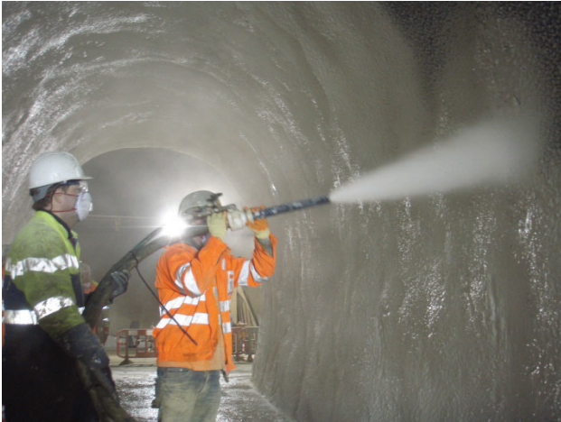
Figure 5: Manual membrane application in cross passages
