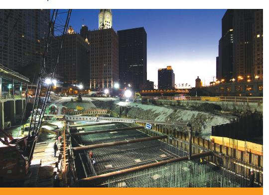
The mat foundation for the Trump International Hotel & Tower in Chicago measured 198 ft (60 m) in length, 60 ft (18 m) in width and 10 ft (3 m) in depth, and required approximately 5,000 yd³ (3,800 m³) of concrete. The designers opted to use self-consolidating concrete (SCC) following the successful use of this technology during construction of the Burj Khalifa building in Dubai.
