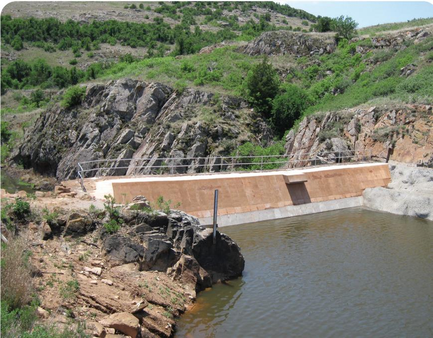
Ketch Lake Dam, built by the landowner Frank Ketch in the 1930's, was built of cobblestone and was a stock pond for cattle. Subsequently, it became a recreational pond. When the dam started giving way in 2010, the Army Corps of Engineers decided to build a new dam directly behind the existing dam. The new dam is 36 feet (11 m) high, 140 feet (43 m) wide and 6 feet (1.8 m) thick at the top and 80 feet (24 m) wide and 20 feet (6 m) thick at the bottom.
